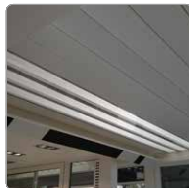
Bringing in light with an extension to a residence
